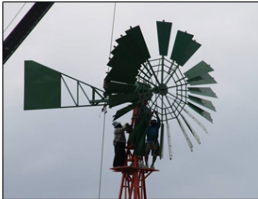
Figure 1(c). Multi-blade wind turbine onsite installation
