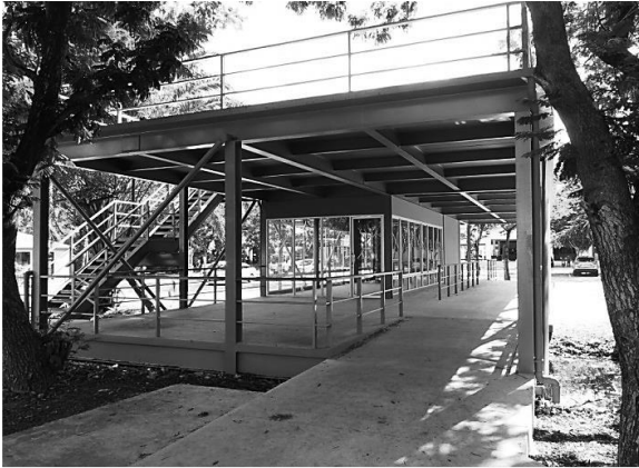
Fig. 11 Welded steel structure
